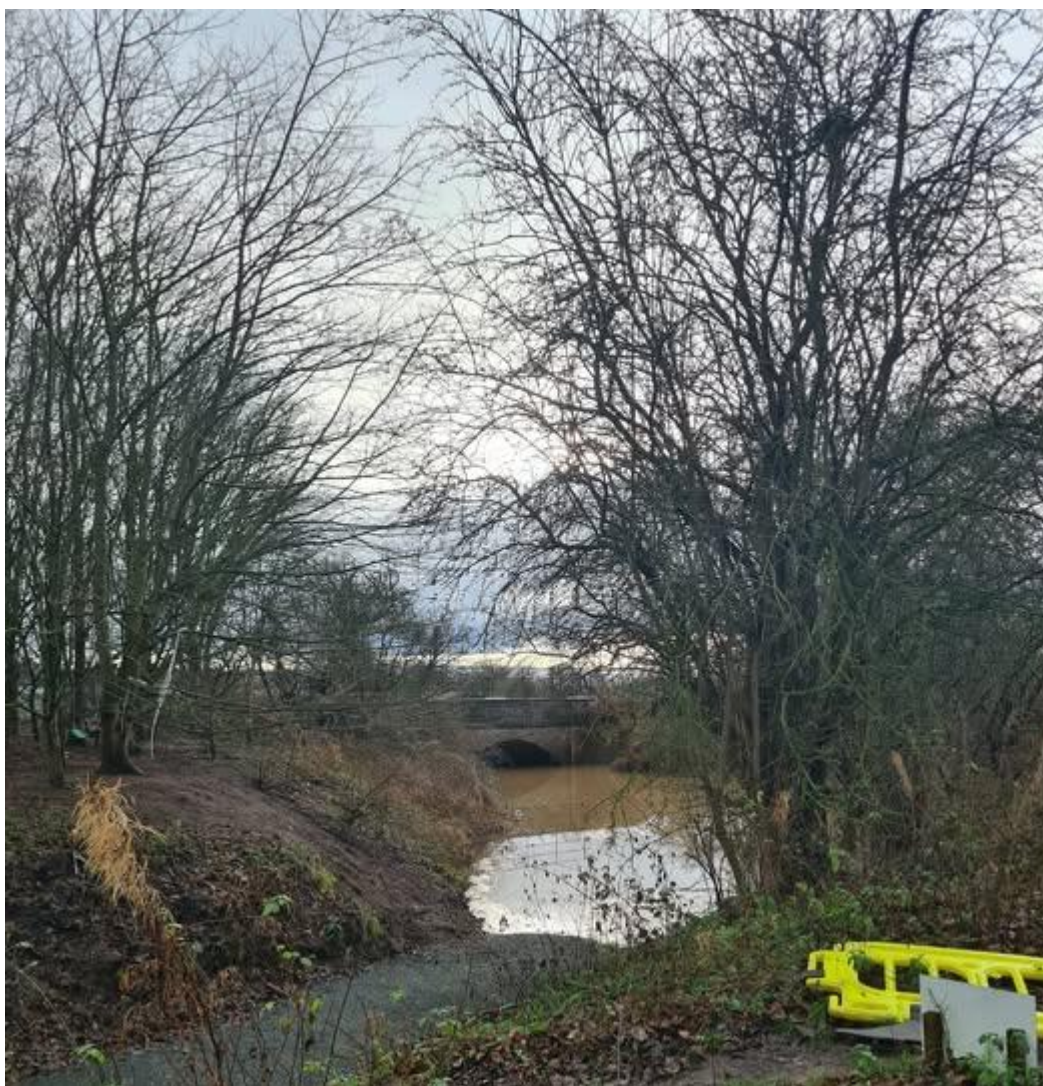
Photograph 3 - Watercourse by railway bridge Allscott - Jan 2024
