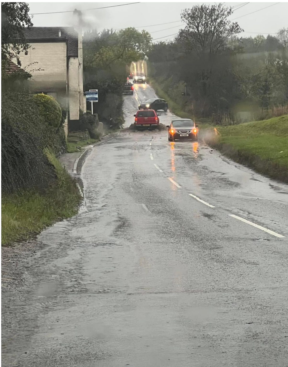
Photograph 6 - Surface water and debris on village road Allscott - Oct 2023
