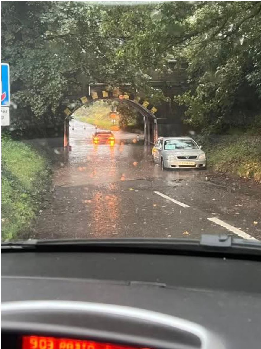
Photograph 5 - Flooded railway underbridge towards Admaston - Oct 2023
